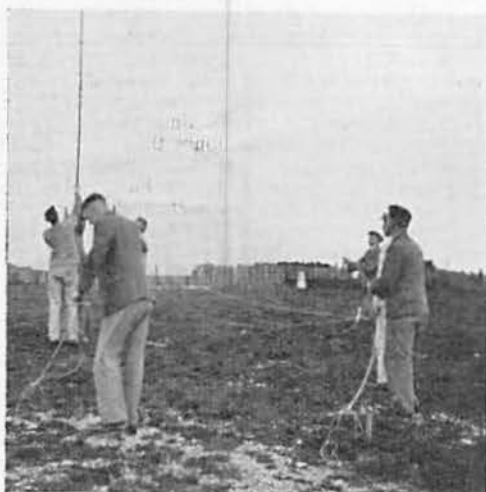
Erecting the mast at District 6 "B" station. GSQA in foreground and G6RP keeping it in the vertical.
